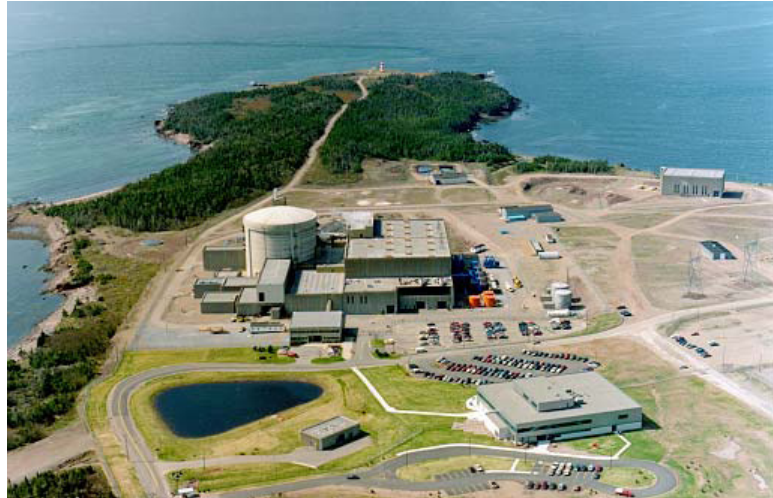
Point Lepreau Generating Station, New Brunswick, Canada
